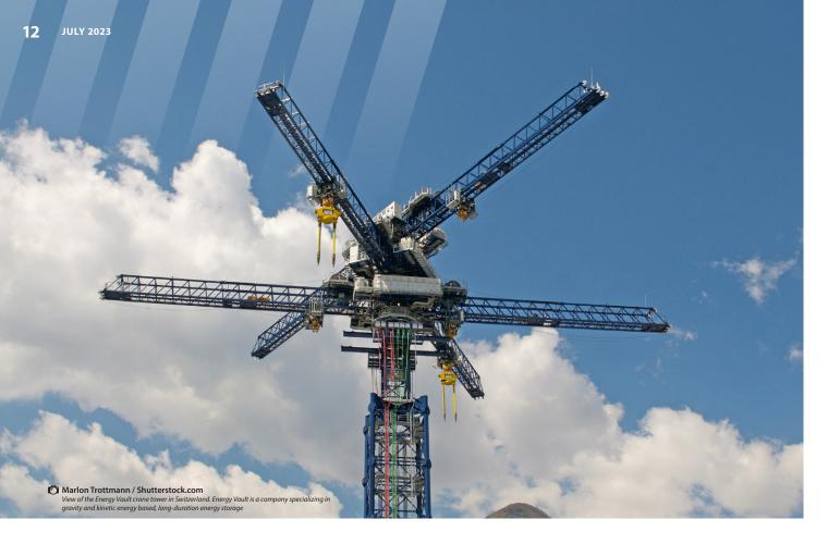
• GES has a high energy density; it has the potential to store a lot of energy in a small area. These systems are also ideal for long-term storage since the gravitational potential energy suffers no losses once a mass is lifted. And since these systems are literally as simple as lifting and lowering mass, they can run continuously and have minimal environmental impact—certainly a desirable alternative to conventional chemical batteries for many power plant operators.
